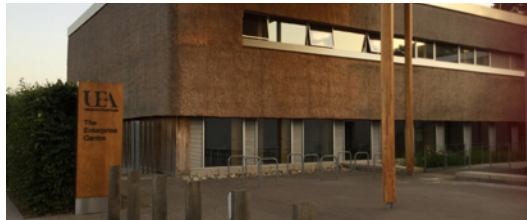
The Enterprise Centre, Passivhaus standard
